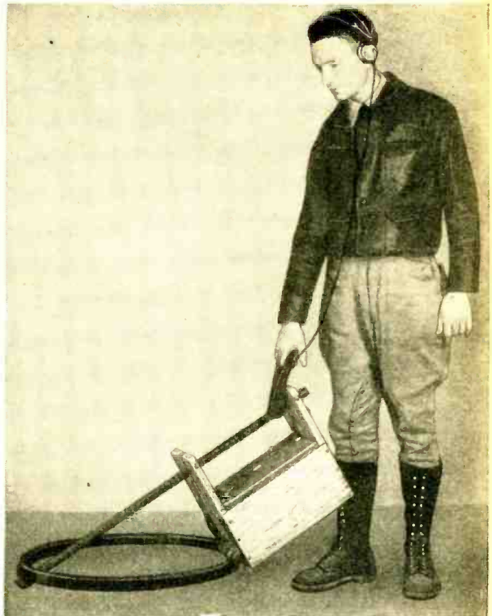
The device in the hands of the author. Note the distance between the ground and the loop.
